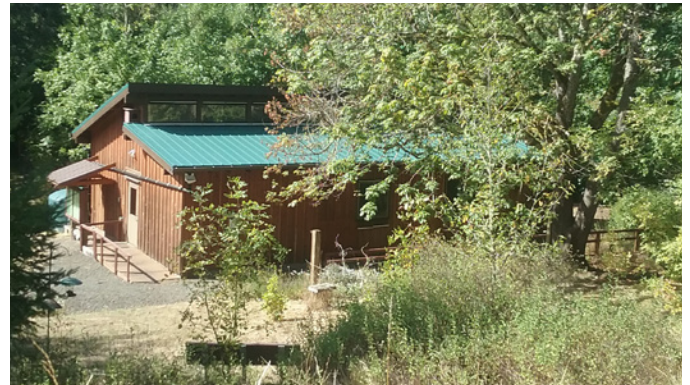
The barn at Hesthavn has a new roof.
